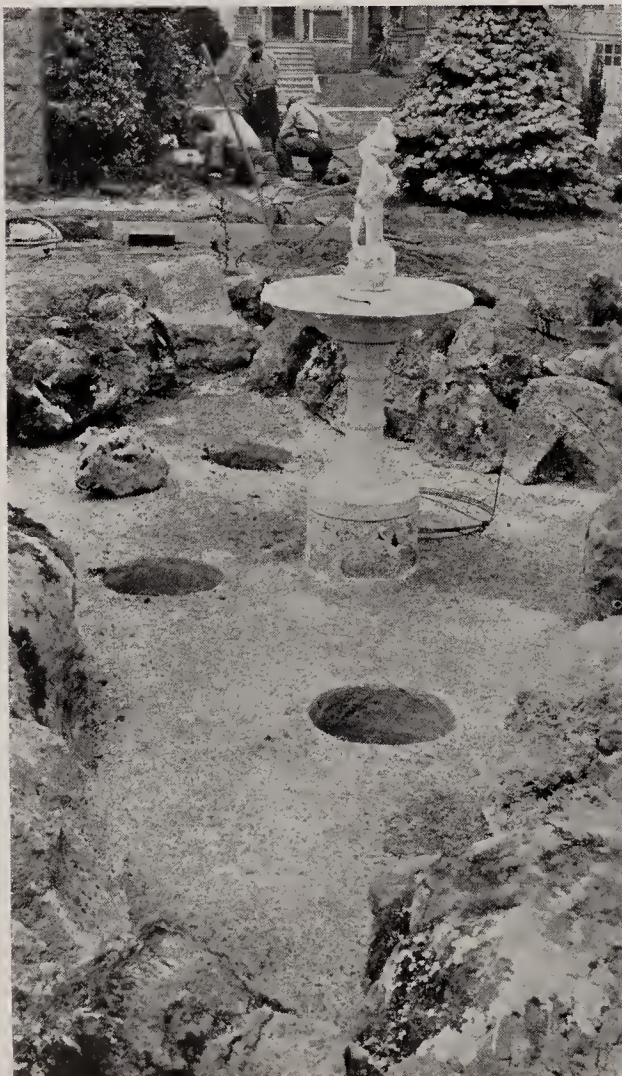
Construction details of lily pool before completion
